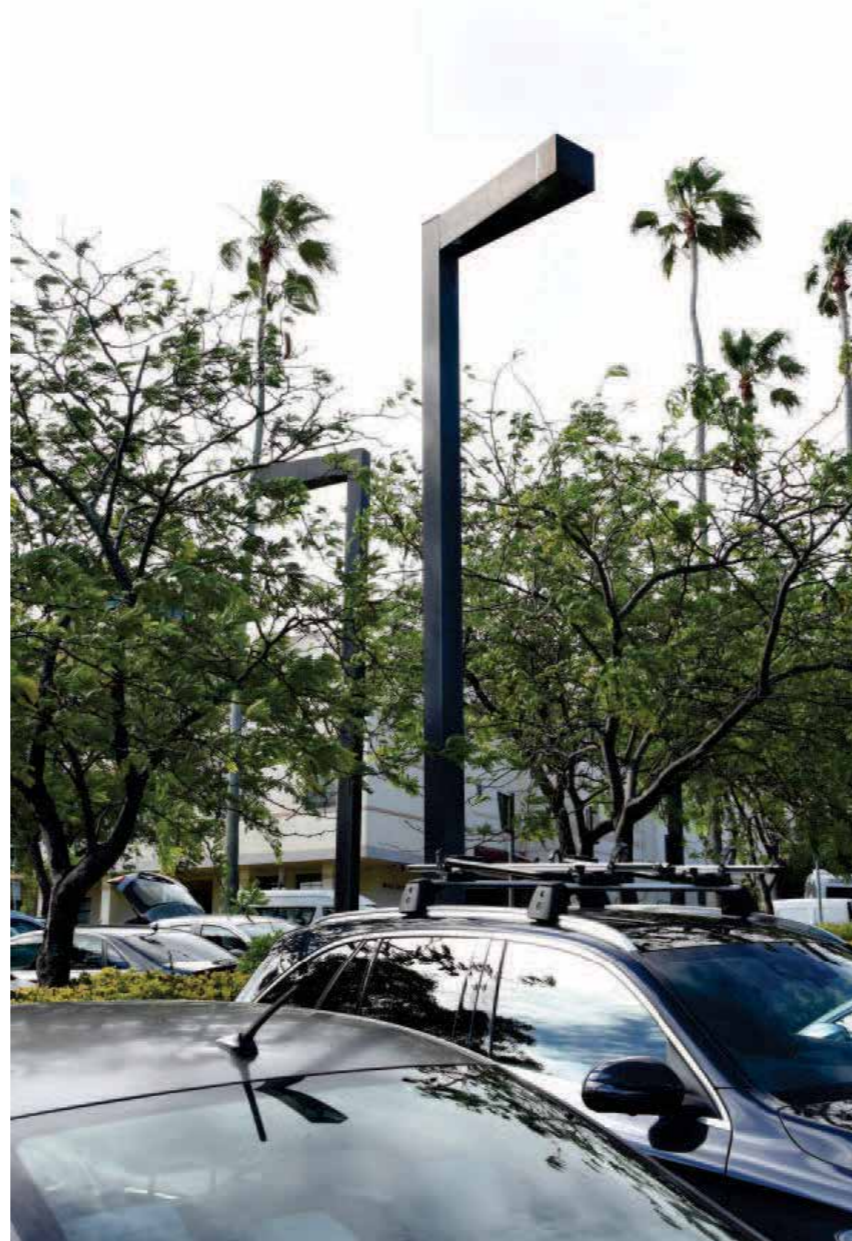
Existing light pole currently used in Mosman
