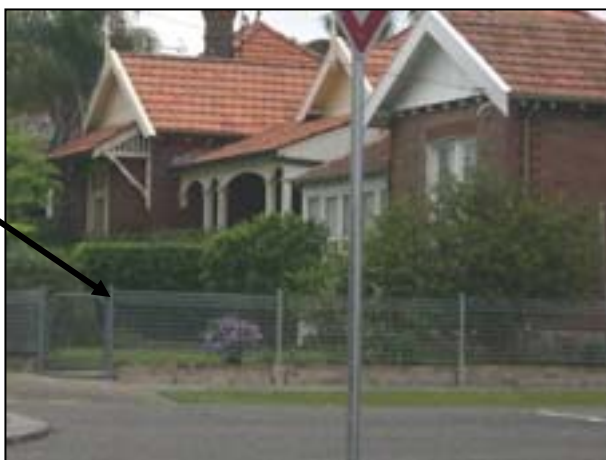
Intrusive Fence of Welded Steel Mesh
