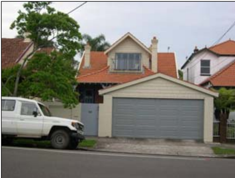
Dormer addition with uncharacteristic and intrusive proportions. Site also features large intrusive garage.
