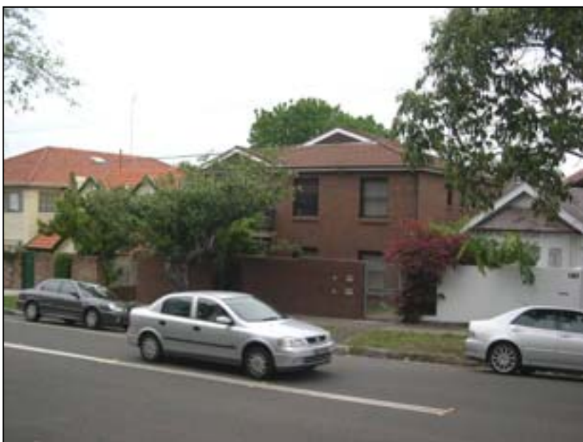
Intrusive 1960/70s infill that is out of scale with surrounding dwellings and its bulk is intrusive to the streetscape.
