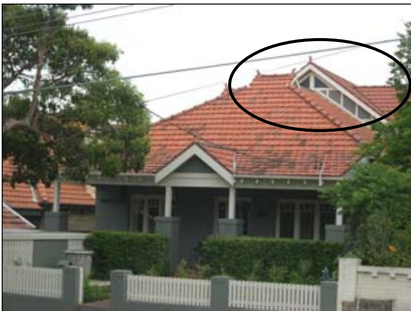
Although original façade fabric has been altered the rear additions are sympathetic because of their setback, scale, sympathetic form and materials. Due to the slope of the site they probably allow two levels at the rear without having impact on the streetscape.
