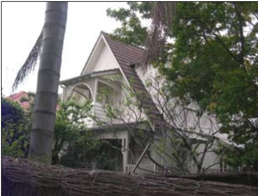
Interesting example of a Federation Arts and Crafts residence on Cabramatta Road with steeply pitched roof, original eyelid dormers and roughcast render walling.
