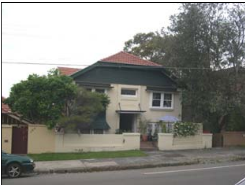
One of the Inter War walk-up flat buildings in Cabramatta Road. Substantially intact featuring detailing typical of the period.
