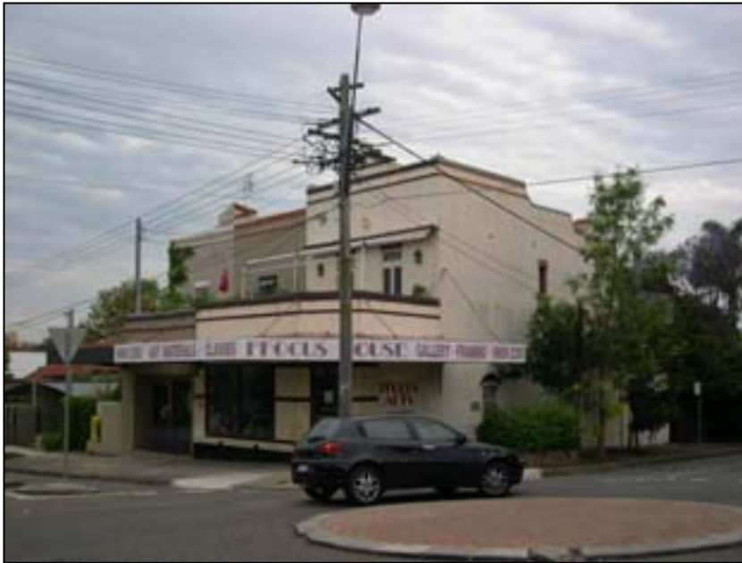
Group of two storey Federation terraces, unusual in the area, with Inter War ground floor addition. Located on the corner of Cabramatta and Bardwell Roads.
