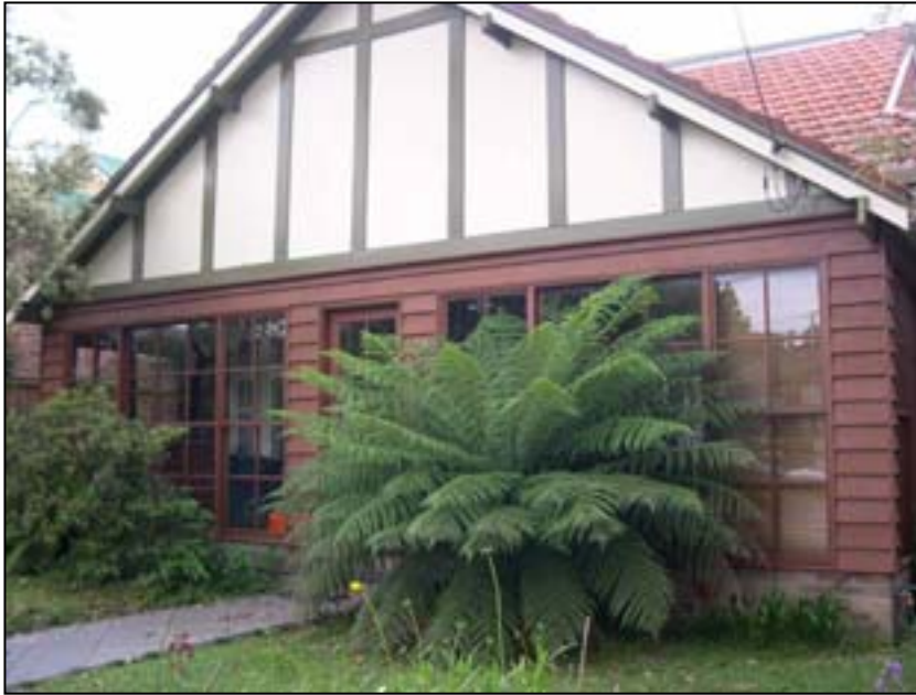
Intrusive enclosure of Verandah of Californian Bungalow. This is reversible as the façade is intact behind.
